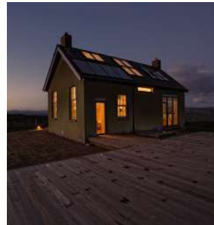
THE CONVERSION OF MONEENATIEVE NATIONAL SCHOOL, IRELAND
